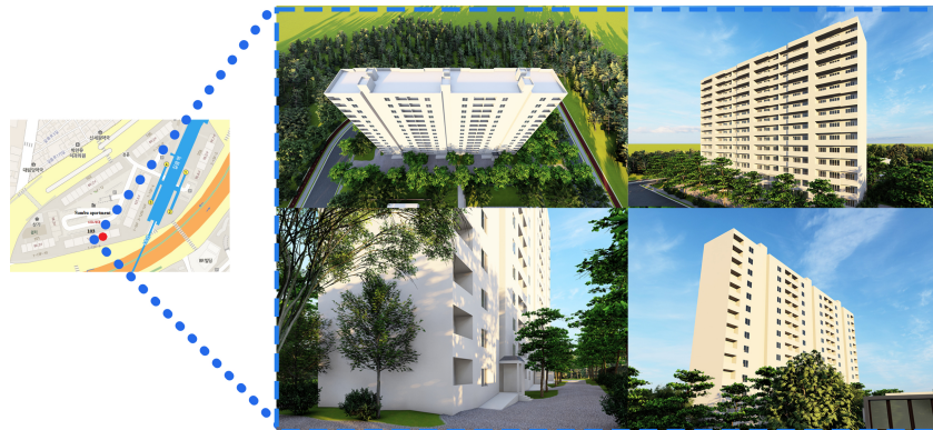
Figure 7. Location of Building 103 in Sambu building complex, Gireum district, Seoul, South Korea.
